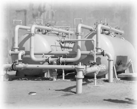
*The Centralia Project conducted by Southern California Water Company is testing a ferric-chloride co-precipitation removal method. Photo Credit: Jason Wen*
