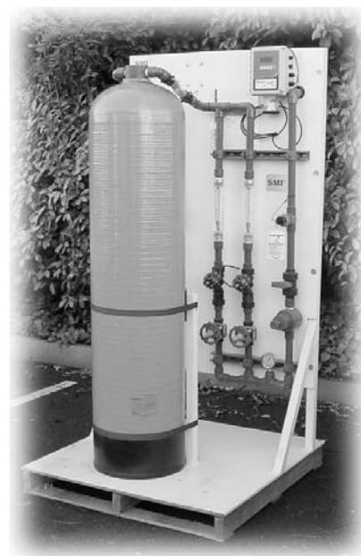
*California Water Services is testing this Sulfur Modified Iron (SMI) unit on a 5-7 gpm side stream from an 800 gpm well. Photo Credit: Dick Wrath*
