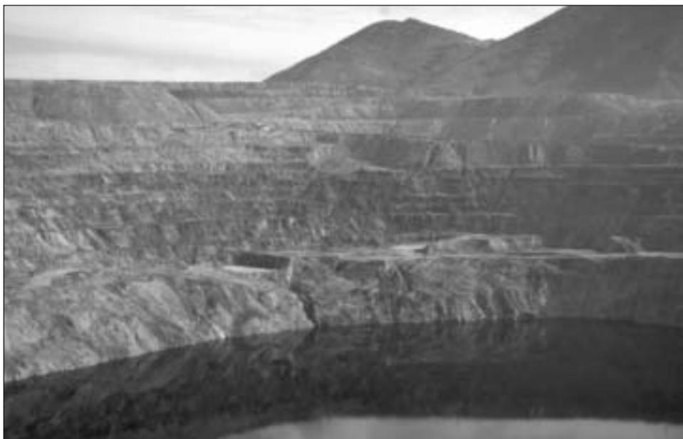
**The Berkeley Pit Lake.** Scientific studies have determined that the Berkeley Pit's water will not pose a threat to human health or to the environment as long as the level stays below the 5,410-foot level. A new \$20 million wastewater treatment plant is expected to be operational by late 2003. For more on the Berkeley Pit, visit [www.pitwatch.org](http://www.pitwatch.org). Photograph by Glenn C. Miller.
