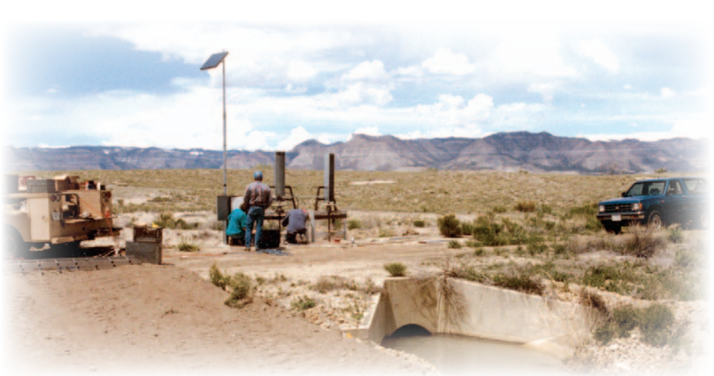
Installing monitoring and control equipment.
