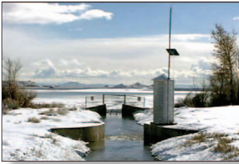
Real-time flow monitoring on Huntington North Inlet Canal.
