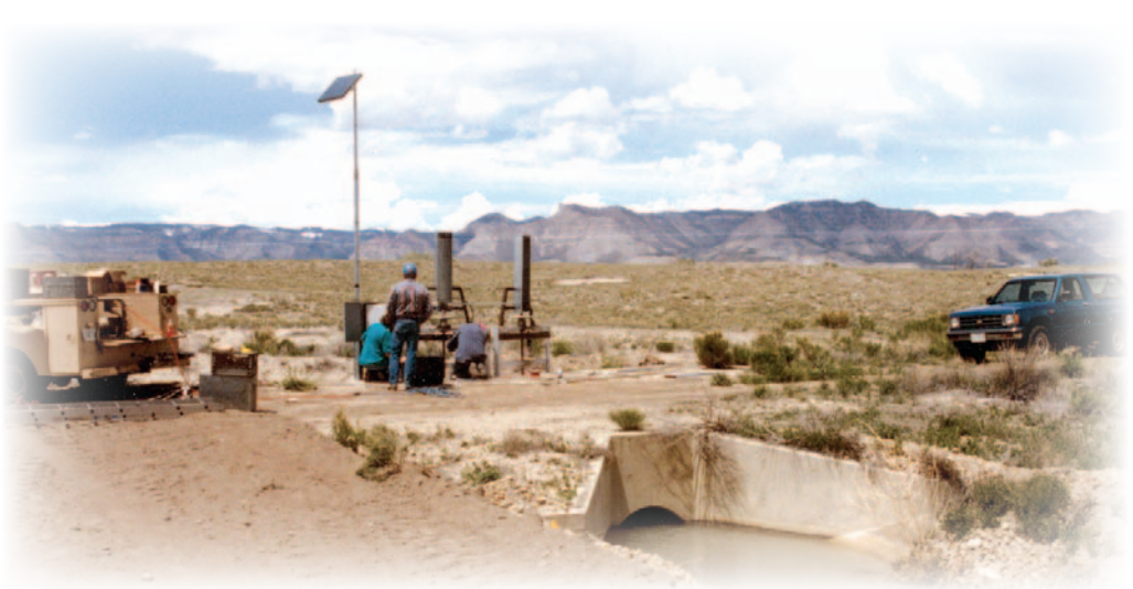
Installing monitoring and control equipment.
