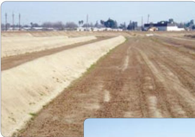
(left) Construction of a recharge basin using the ridge and furrow design. (below) Partially filled basins showing the ridgetops exposed for wave action. Photos by Dennis E. Peyton.
