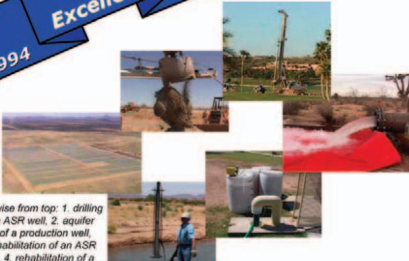
Clockwise from top: 1. drilling of an ASR well, 2. aquifer test of a production well, 3. rehabilitation of an ASR well, 4. rehabilitation of a vadose zone recharge well, 5. full-scale basin recharge, 6. drilling of a vadose zone recharge well.
