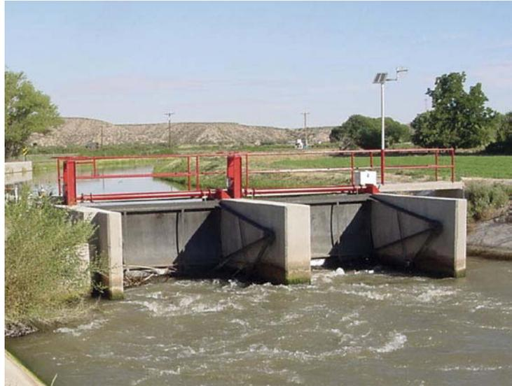
Radial gate check with telemetry.
