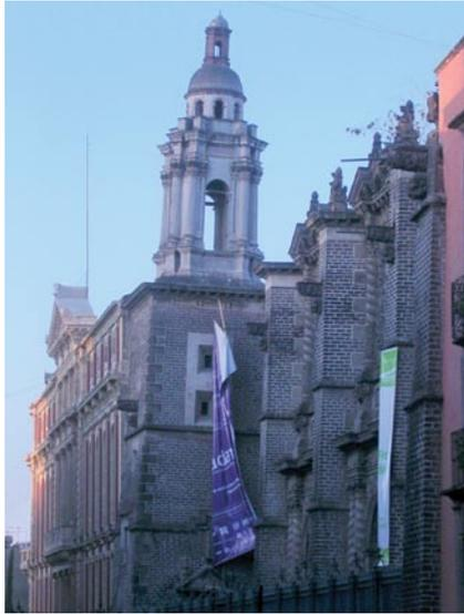
Groundwater overdraft has led to uneven subsidence in Mexico City, as illustrated by the tilted lines of this building.
