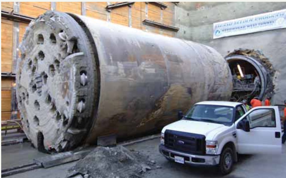
The tunnel-boring machine, shortly after it emerged from the San Bernardino Mountains.
