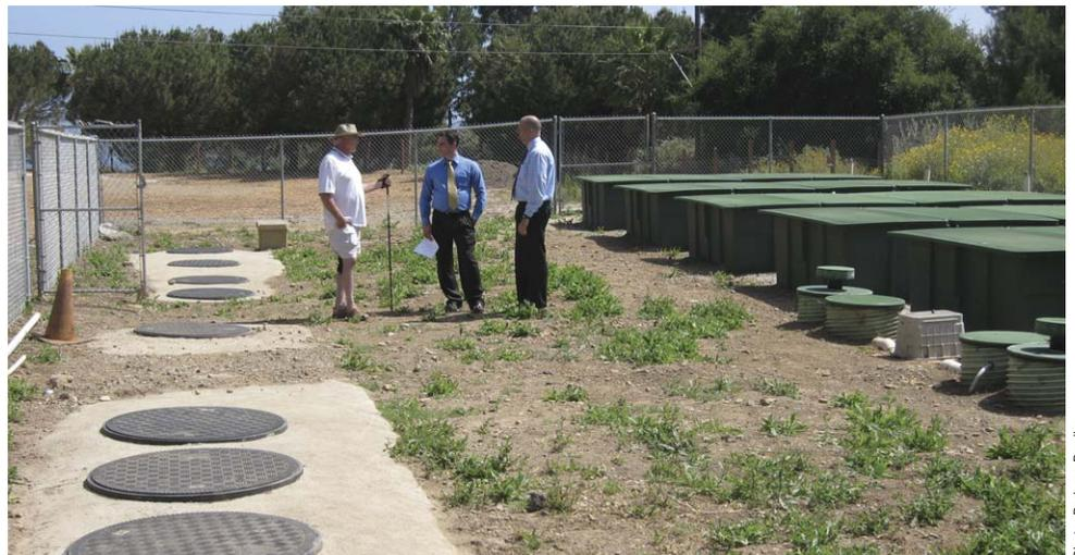
An onsite wastewater treatment system for a restaurant in Malibu, California; underground treatment tanks are in the foreground and secondary treatment units are on the right. A portion of the treated wastewater goes to subsurface drip irrigation in a green belt.
