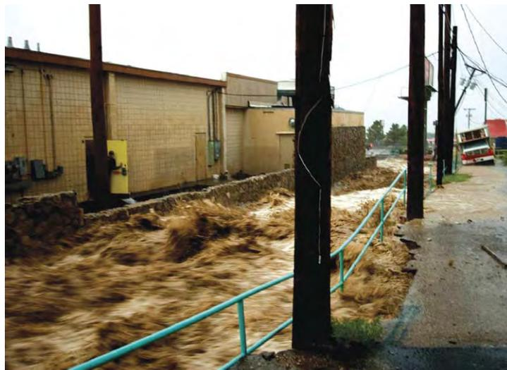
Upscale arroyo-side development (left) and flood damage due to deficient arroyo drainage system (right) on the west side of El Paso.
